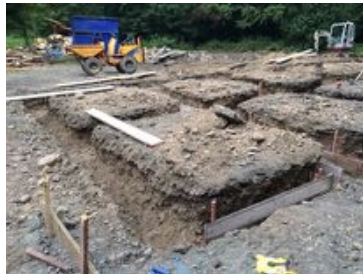
The foundations of the new hut
